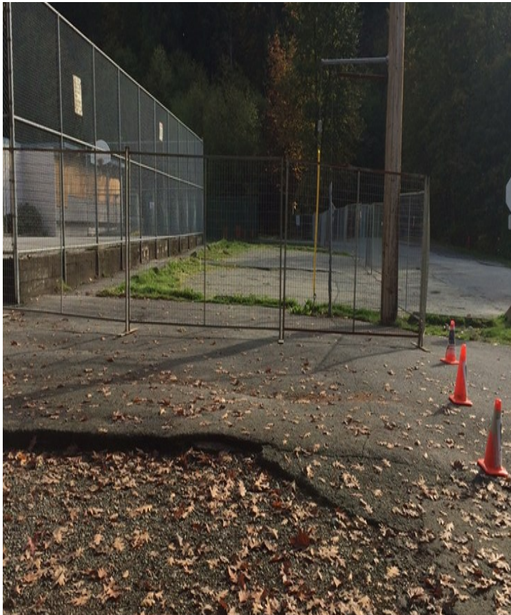
Construction zone fencing
